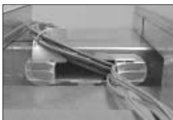
Bend Radius control for communication cables.
